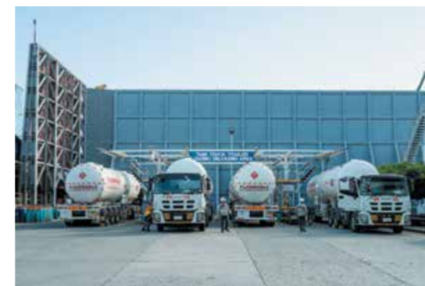
The new LPG refilling equipment in our Gasul Terminal in Pasig is one of several projects completed in support of our LPG business growth.
