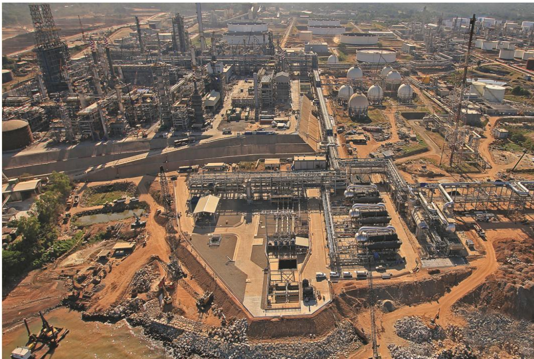
Petron’s US$ 2-billion Refinery Master Plan Phase 2 (RMP-2) consists of 19 units.
